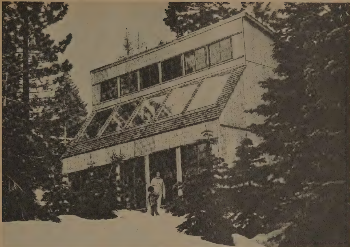
The Kubota/Smith Solar House at 7,000 feet, near Lake Tahoe. Snowing at nine in the morning with 5 feet of snow on the ground. Toasty inside.
